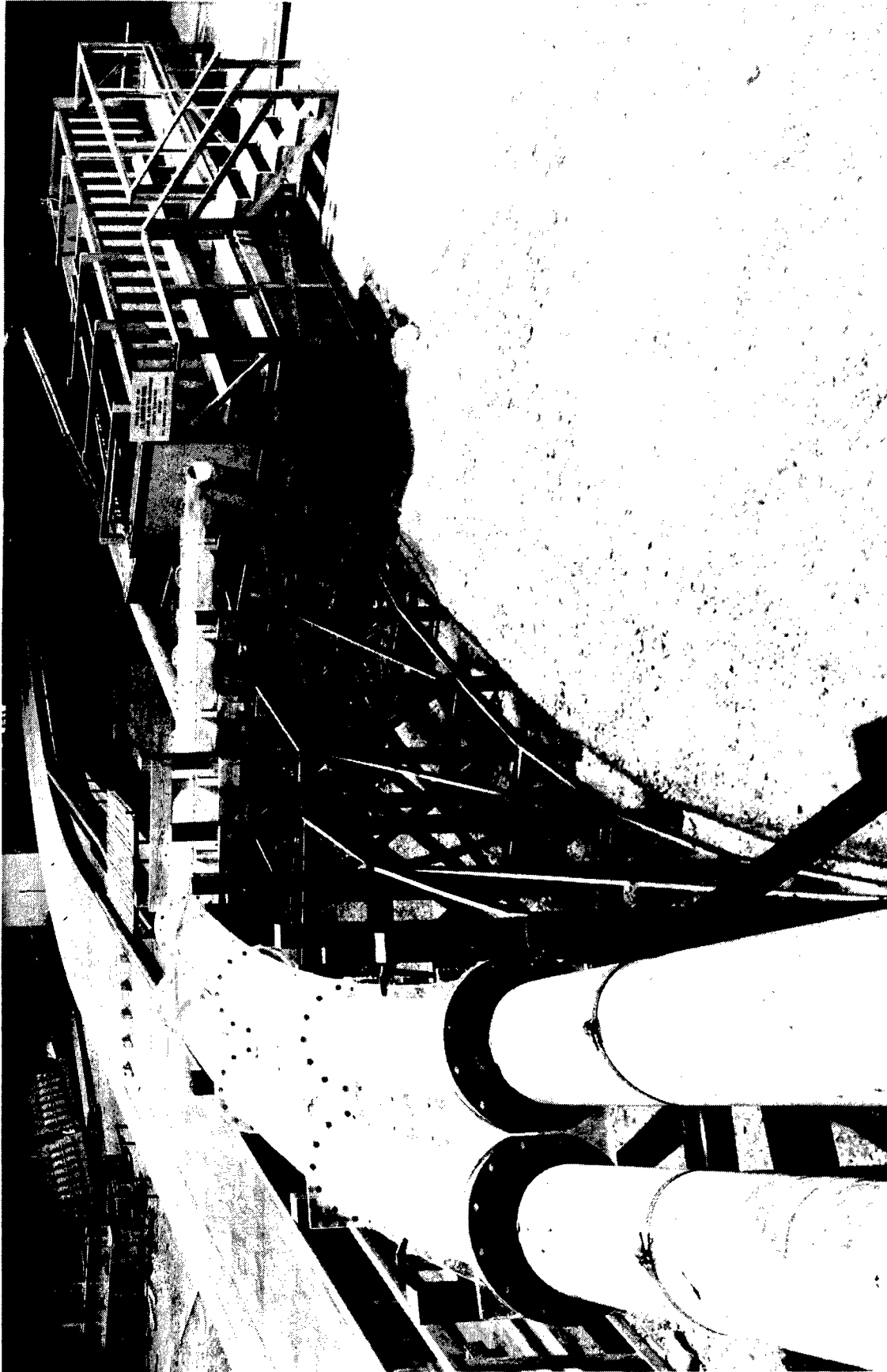
a. Looking downstream at the two 54-in.-diam conduits and the basin for the fish and flow flumes
