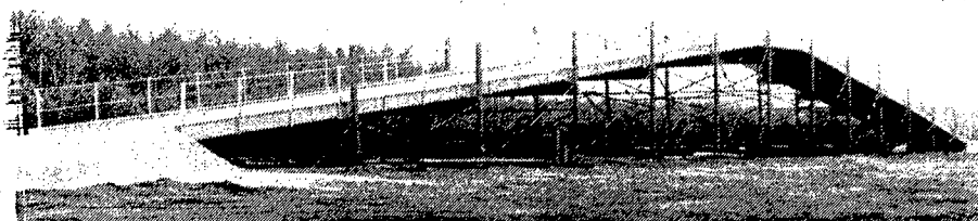
Figure 5. Overpass Structure With Vertically Adjustable Supports
