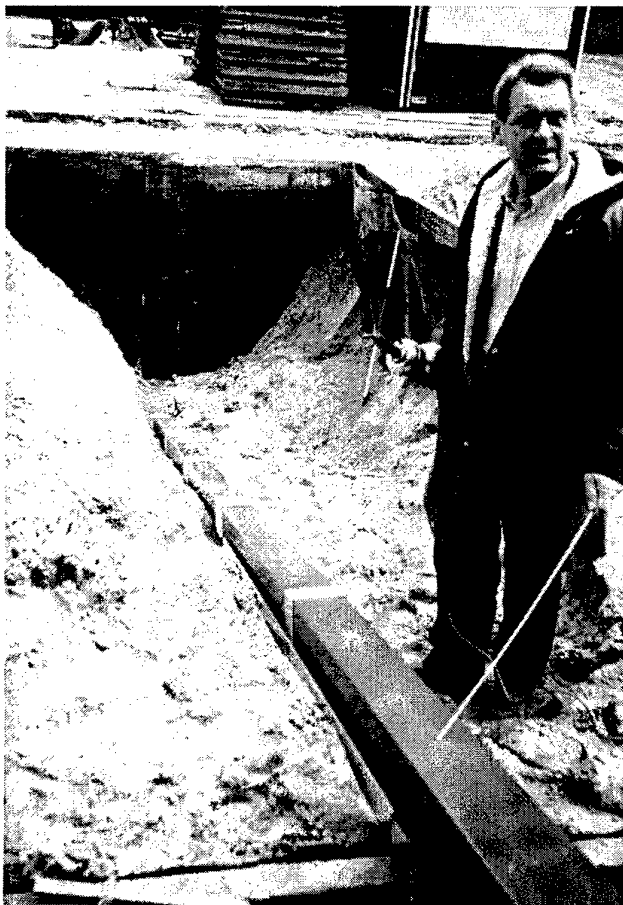
Figure 3.12 Installation of a square PVC tube running from the surface of one side to the bottom of the other side of the box, facilitating measurements of EM transmissions into the ground.
