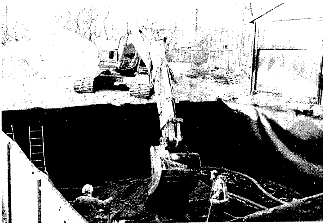
Figure 3.10 Overview photo. The wooden box is now ready to be filled with sand.
