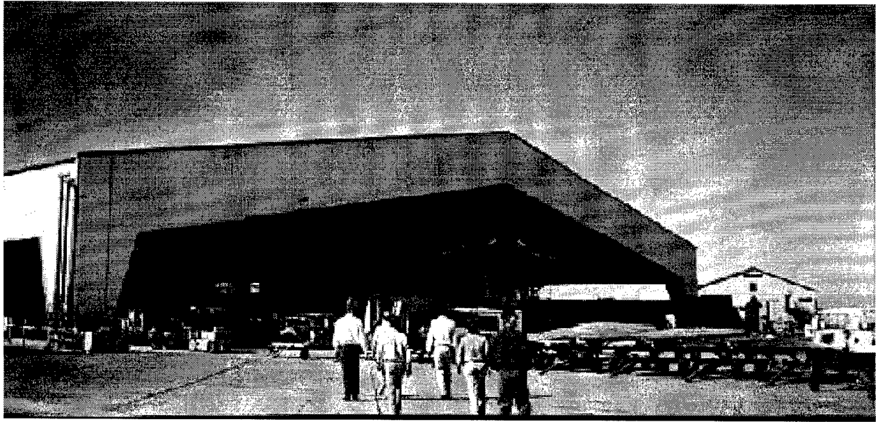
Figure 1. Aircraft Repainting Facility at McClellan AFB
