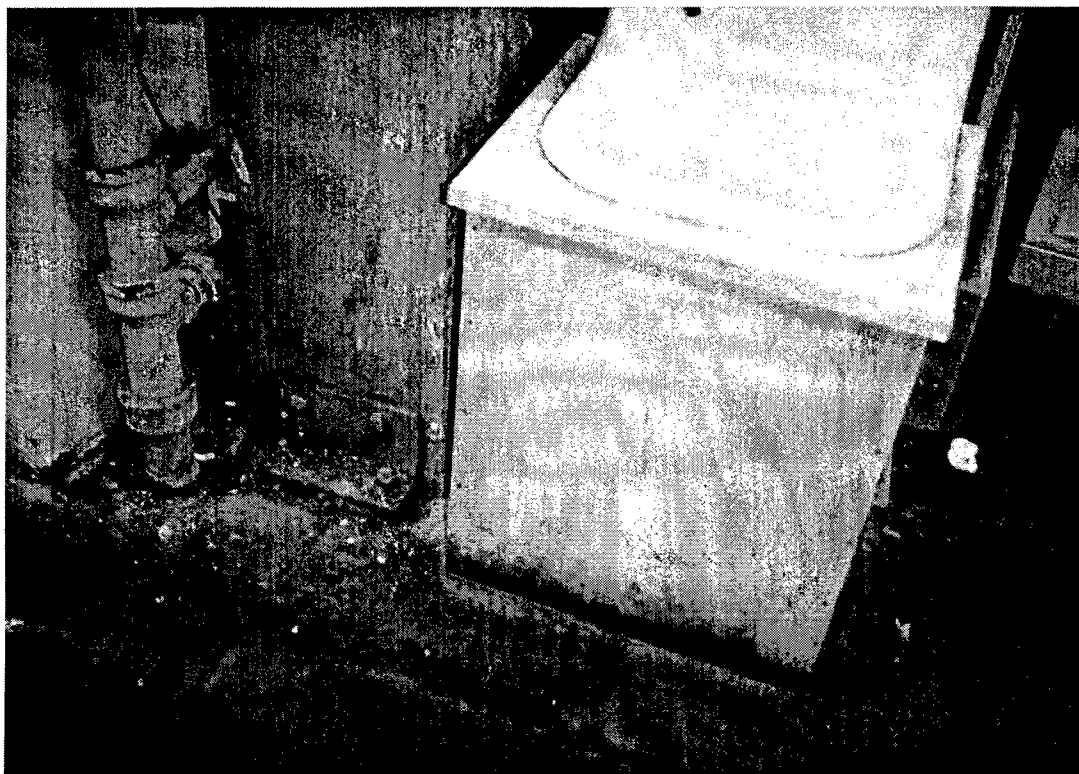
Photo 25. Leakage from a sink that will damage a column.
