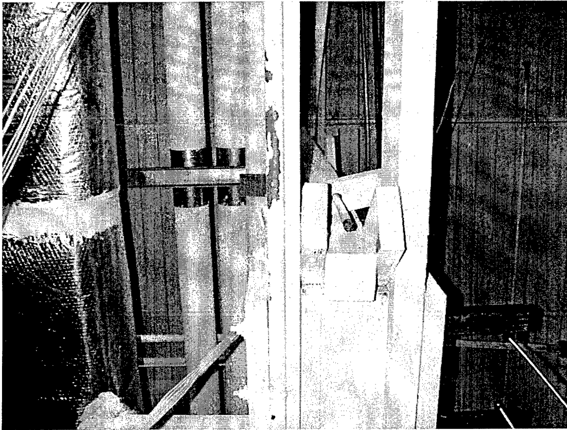
Photo 18. Cantilever pipe support on diagonal members of Truss 34, Area A.
