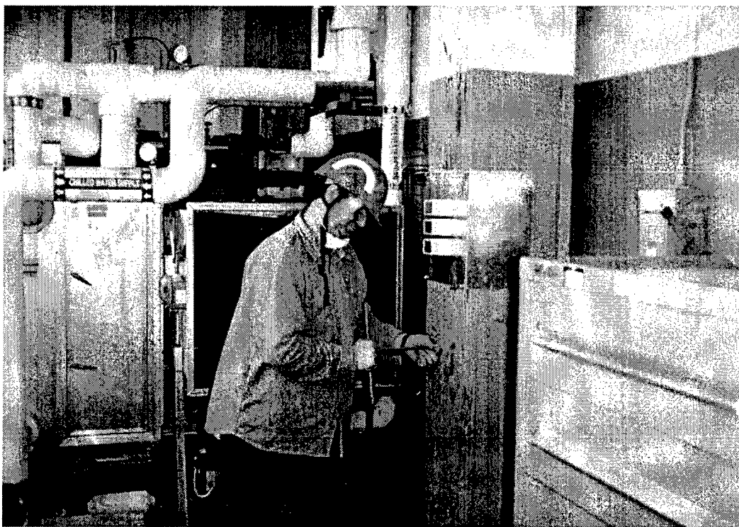
Photo 22. Using the coring on termite damaged column.
