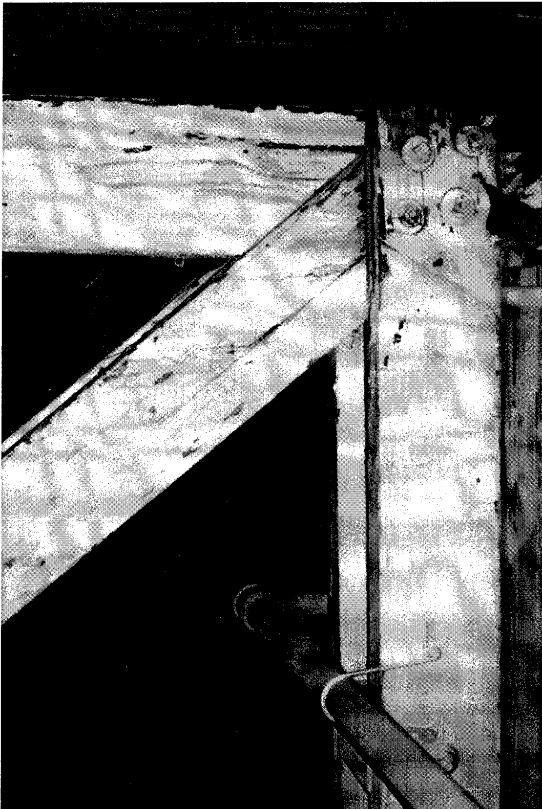
Photo 9. Major damage due to decay in a joint in Area A.
