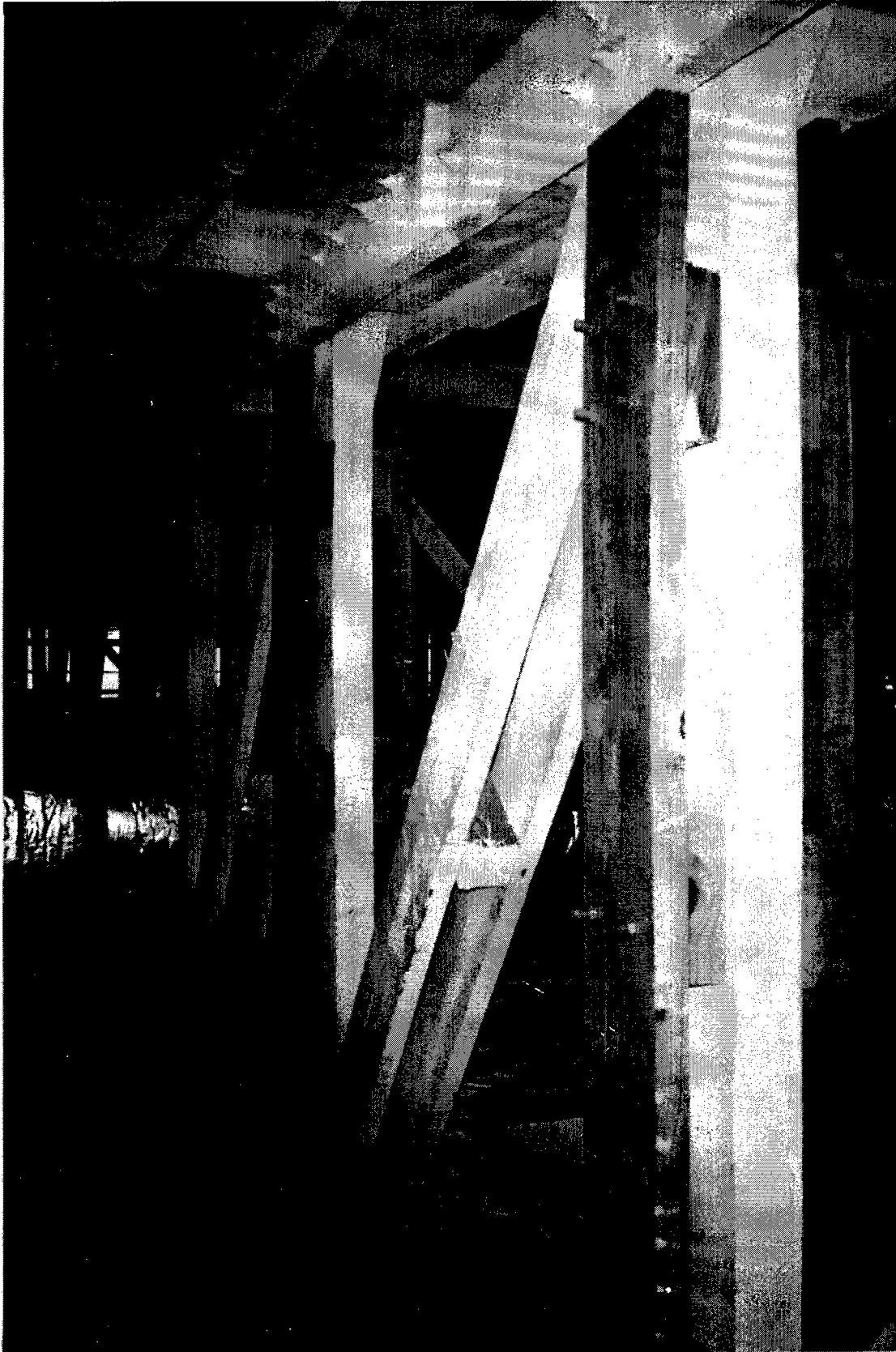
Photo 3. Typical type of existing repair in Area A.
