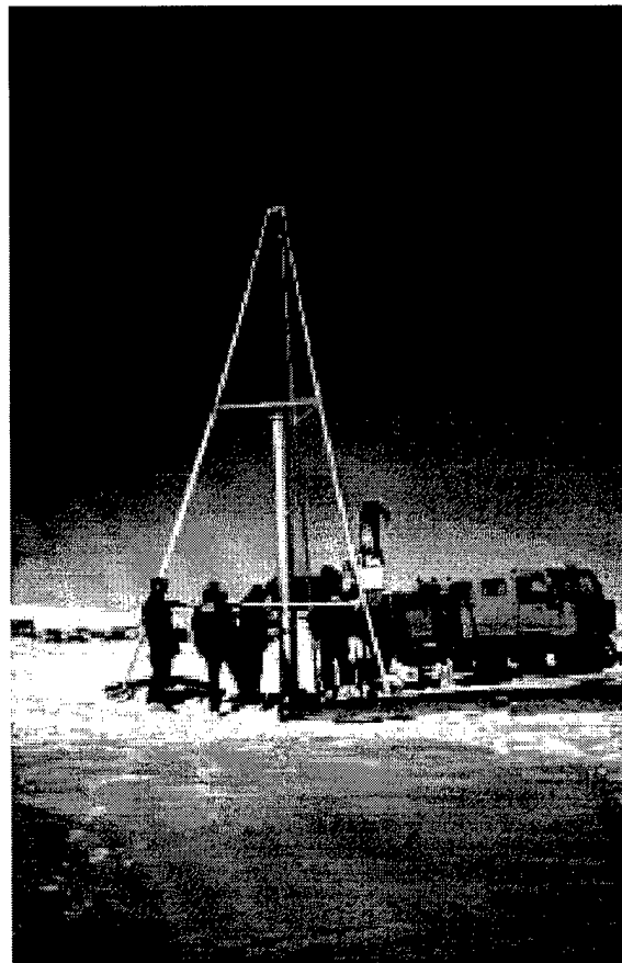
Figure 14. Installing vertical chip conveyance tubes.
