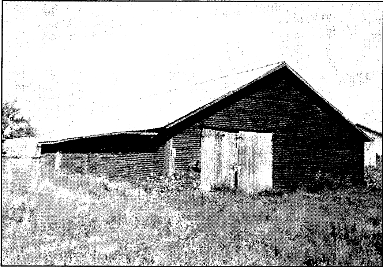
Figure 17. Structure D (Frame Barn), south and east faces.
