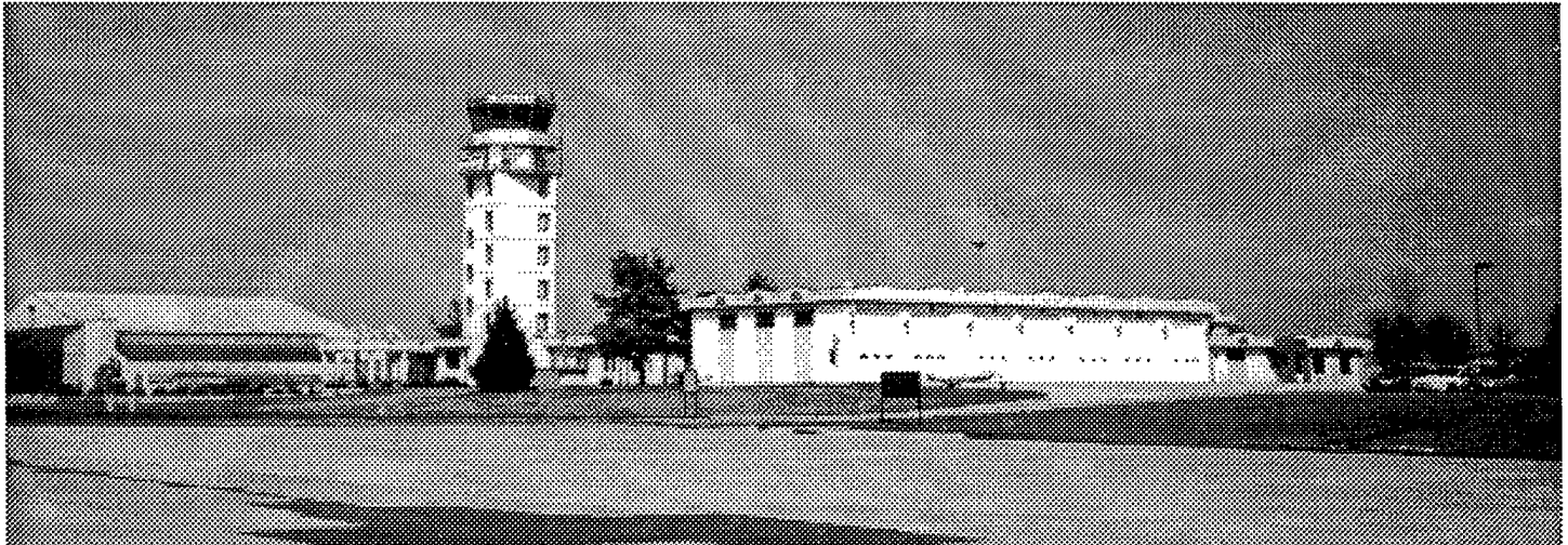
Air traffic control tower, parking area, and hangars.
