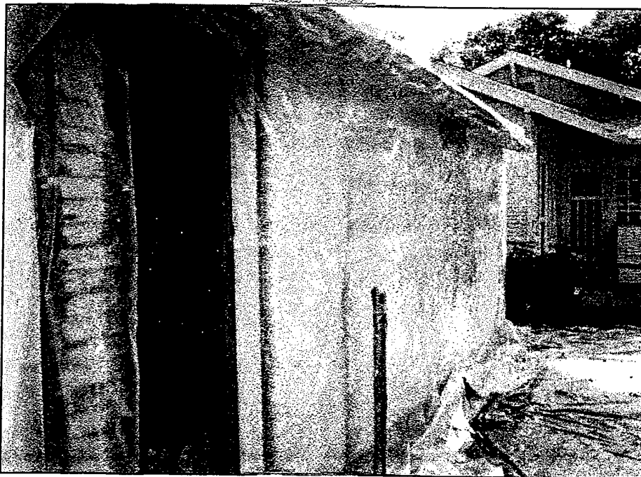
Figure 4. Containment for Chemical Stripping on Building 139
