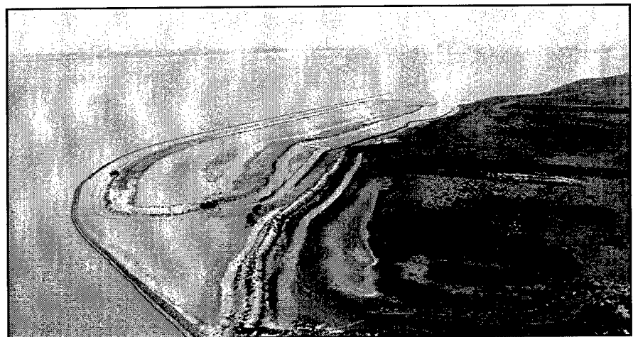
Figure 1. Newly constructed marsh requiring breakwater to dissipate wave energy; the breakwater is visible from just left of the bottom center, stretching to the left and arcing around the newly constructed marsh
