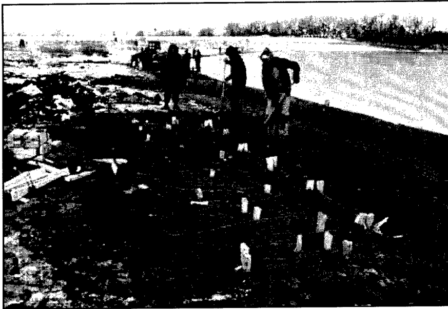
Figure 2. Breakwater made from a coir geotextile roll with workshop participants installing a brush mattress made from willow
