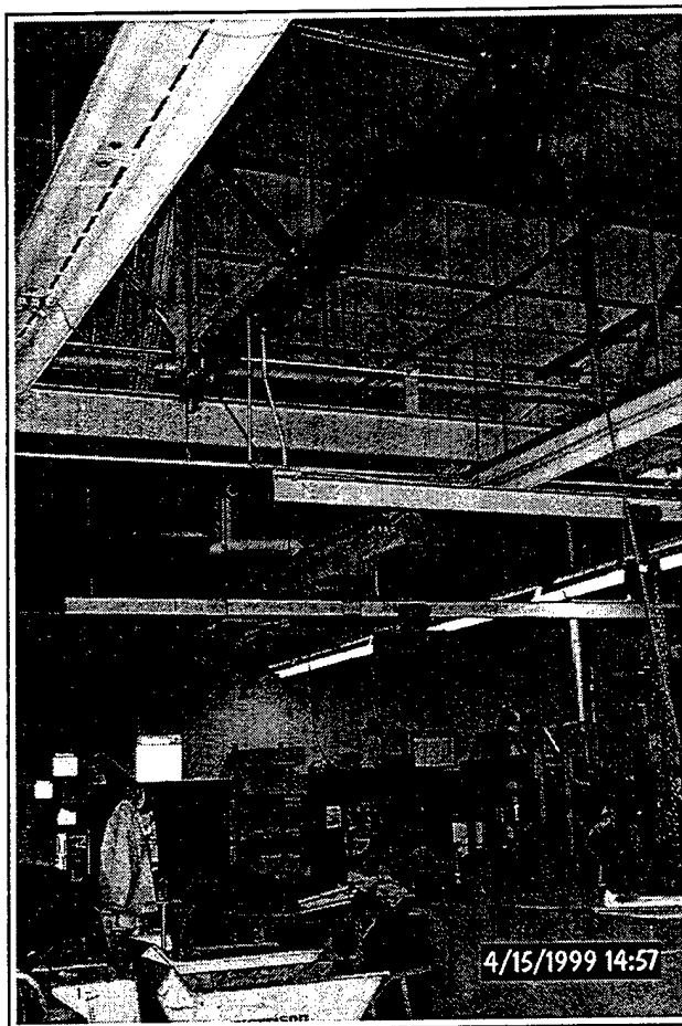
Figure 1. North warehouse lighting.
