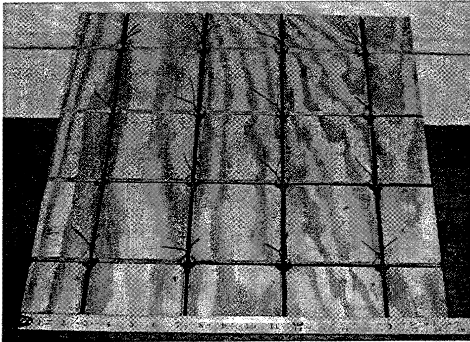
Figure 1. Photograph of One Layer of Reinforcement During Assembly.
