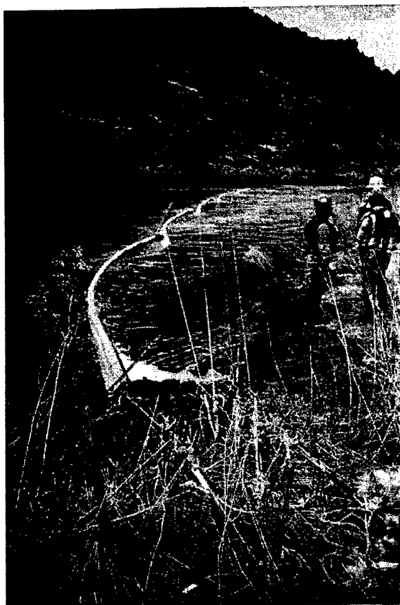
Figure 12. Cascade Booming of a Narrow River
