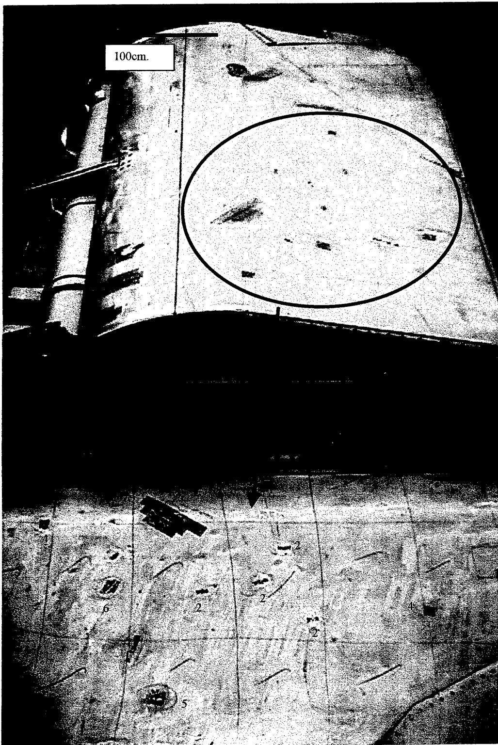
Figure 7.0 An example of the potential number of injection repairs, which may be associated with one F-111 honeycomb bonded component. Injection repair hole numbers are indicated. None of these repairs had been protected with a structural patch.
