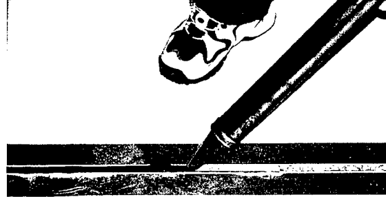
Round closed cell polyethylene backed rod. Bulk chalking gun.
