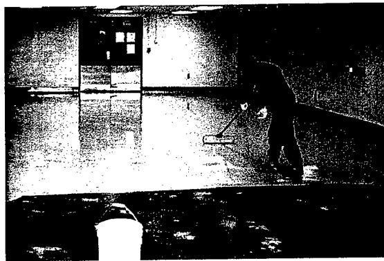
Application of topcoat.
