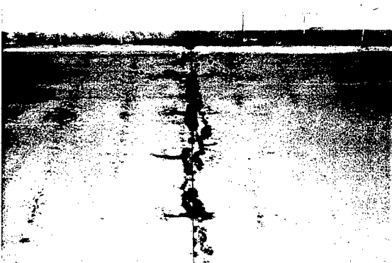
Shot blasted surface with skydrol saturated construction joint (Dark color).
