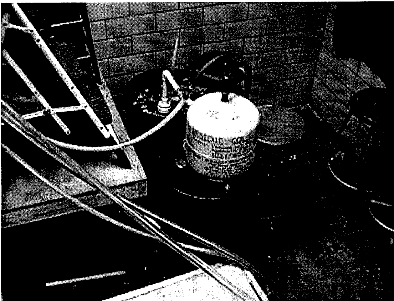
Fig – 4 High Pressure Moisture Collection Tank
