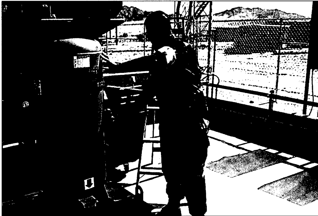
Figure A-6 Ensure main air line valve is in the "OPEN" position. Open valve below compressor tank to drain water. Close valve when complete. Note! Avoid touching copper tubing on side of compressor.
