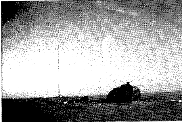
Cause: Aircraft struck tower at night.
