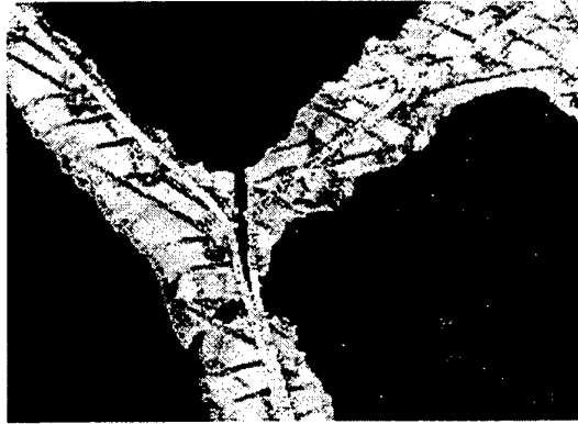
Figure 15. Cracking through the skin to core fillet and into the node bond in a direct moisture ingress sample after 16 weeks exposure.
