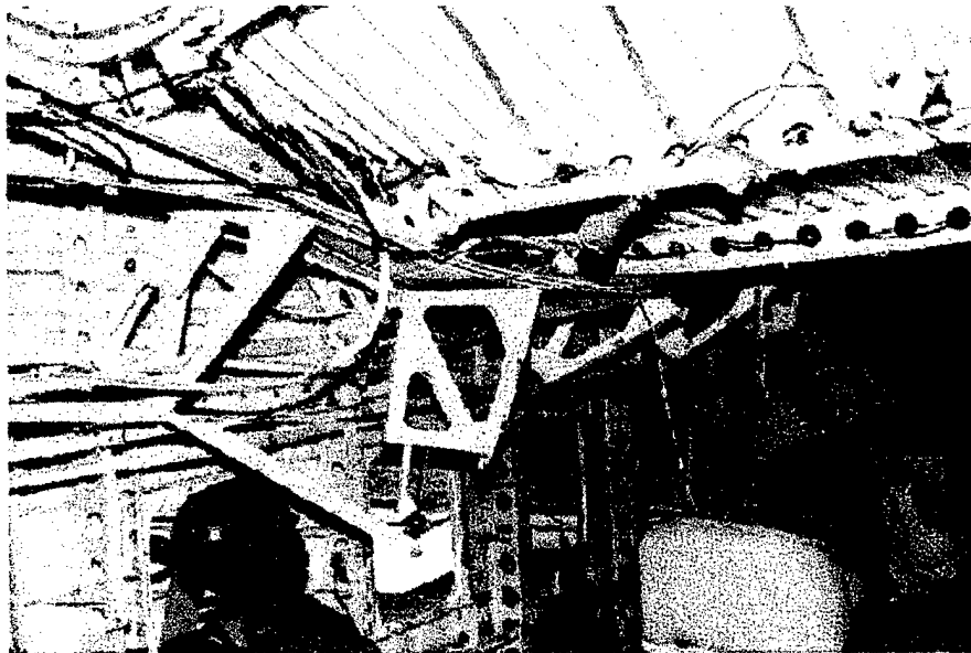
FIGURE 33. CEILING DEFORMATION POSTTEST PILOT SIDE
