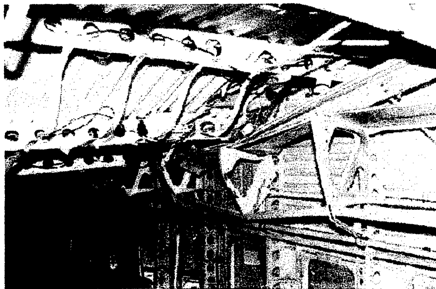
FIGURE 34. CEILING DEFORMATION POSTTEST COPILOT SIDE
