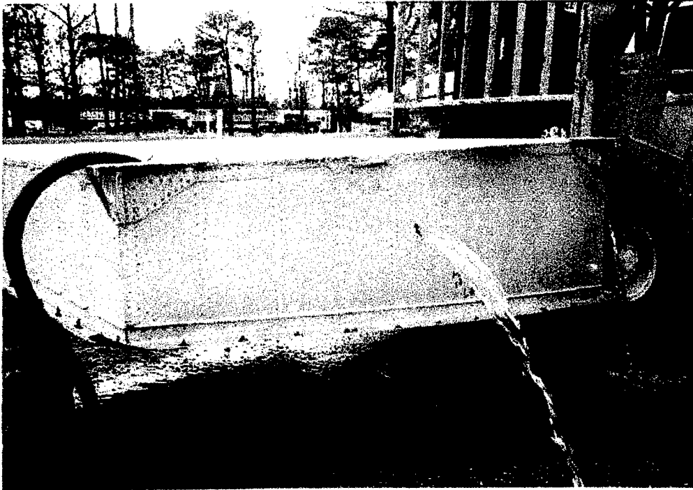
FIGURE 17. CRACK IN CELL 4 PILOT SIDE
