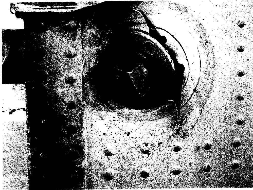
FIGURE 19. CRUSHED GRAVITY FEED OUTLET IN CELL 4
