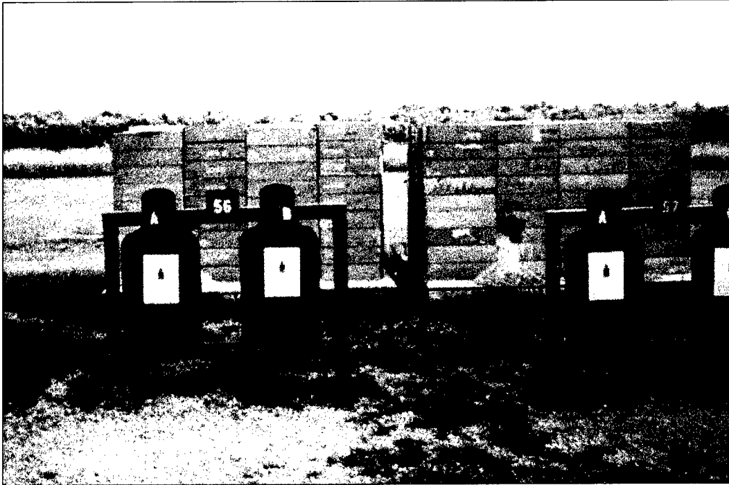
Figure II-2. SACON backstops behind 25-Meter range targets.
