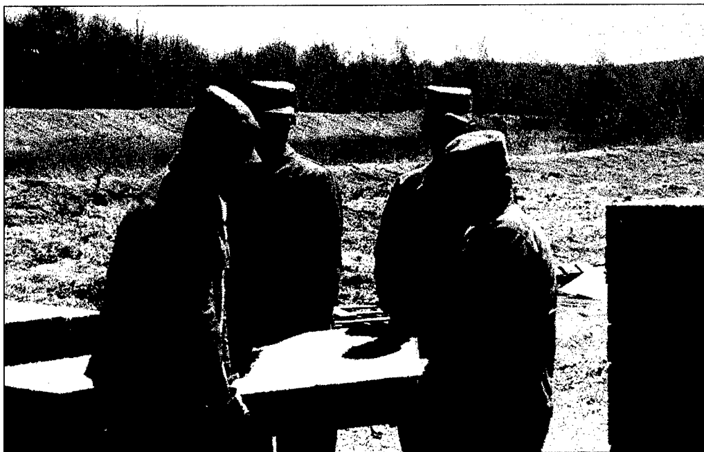
Figure IV-5. Four-man lift - 200-pound SACON block.
