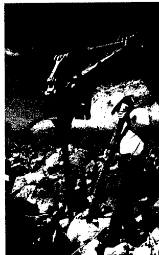
Figure 5. Stinger on backhoe making pilot hole in which to insert a dormant willow post (photo courtesy of Chris Hoag, NRCS)
