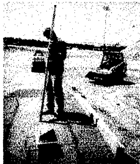
Photograph 7. Base Course Post-Compaction Nuclear Densometer and Rod and Level Measurements
