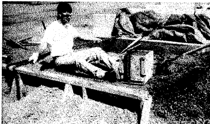
Photograph 10. Undercutting the Clay
