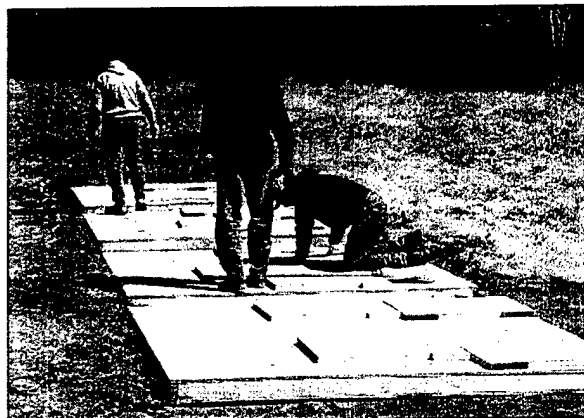
Figure 4-7. Plywood base for walls.
