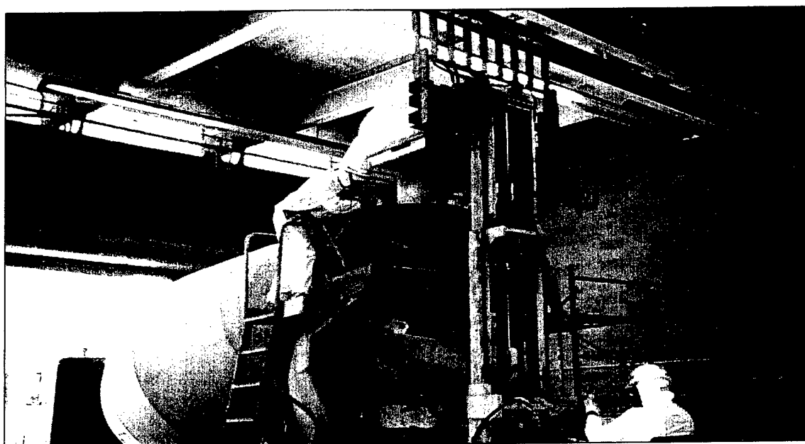
Figure 4-38. Mixing in recycled aggregate.
