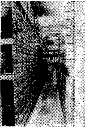
The KAMA multiplex equipment
