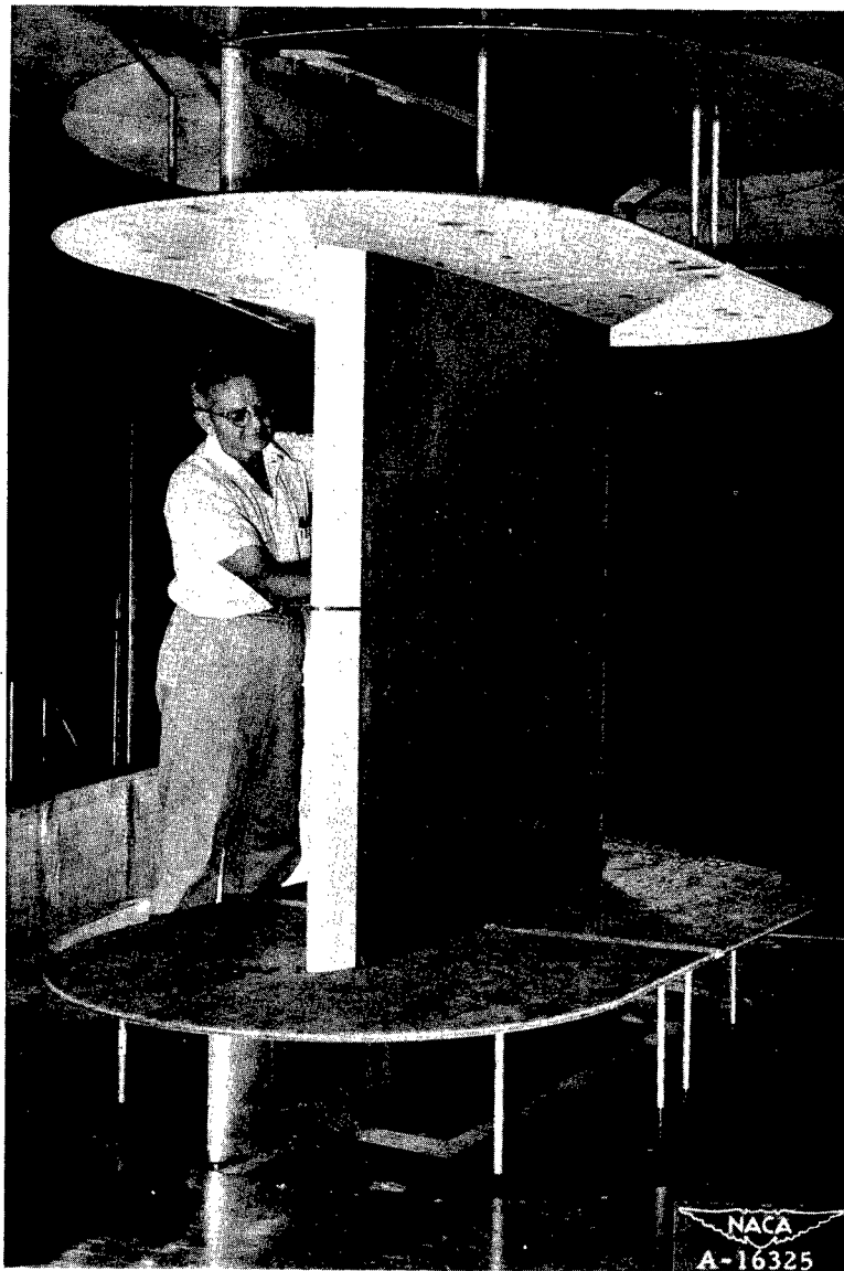
Figure 1.— The 10.51-percent-thick symmetrical airfoil with a porous leading edge.
