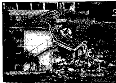
House destroyed in Stolac, Bosnia Source: SFOR.
