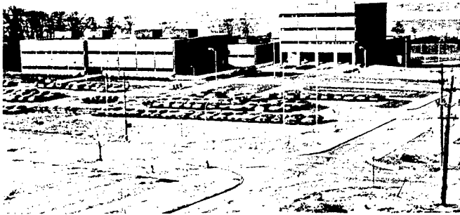
New Materials Laboratory complex under construction
