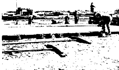
Laying Wright Field's first concrete runways
