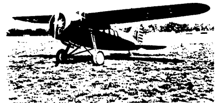
Detroit Y1C-12 had monocoque aluminum fuselage, 1931.
