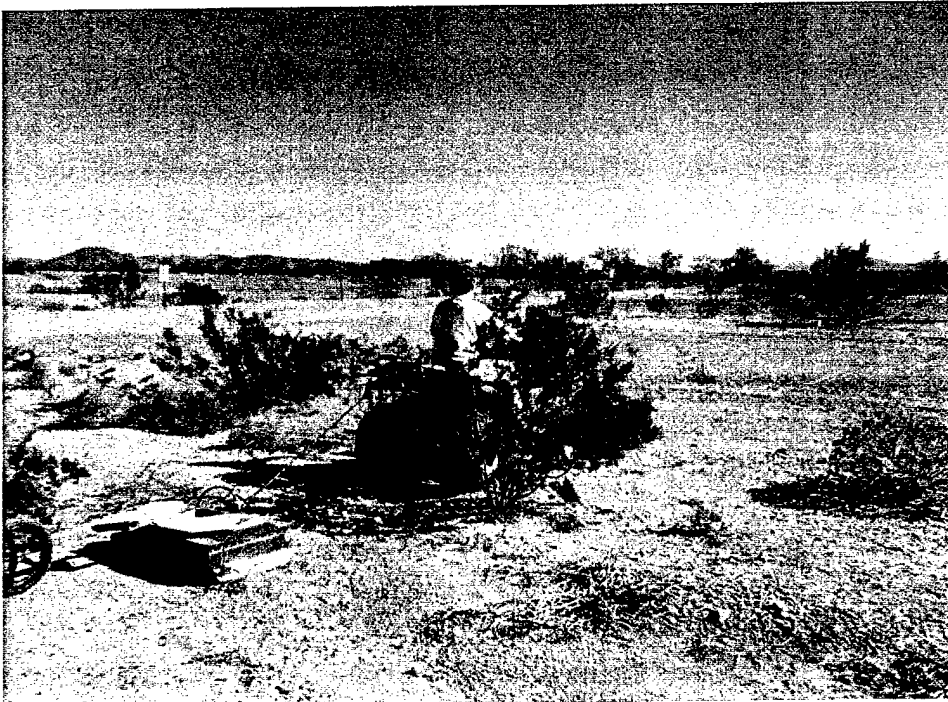
This worker is using ground penetrating radar to perform a survey.
