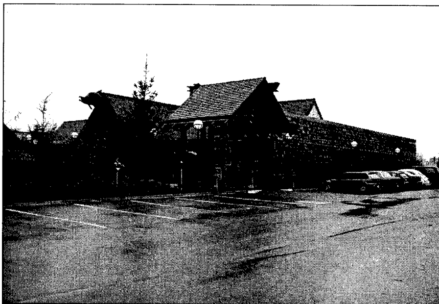
Figure 24. Exterior view of the OSMA in Eugene, Oregon.
