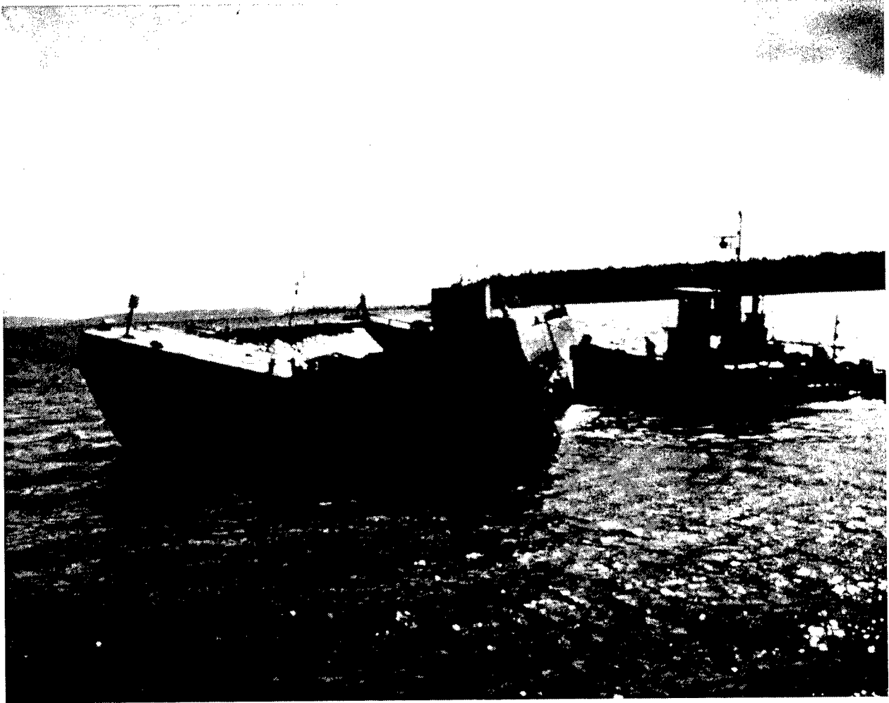
Figure 20. Spreading technique for capping by barge movement
