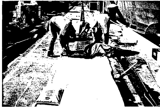
Fig. 20 – Curing a repair. Placement of water saturated, plastic coated burlap over repair.
