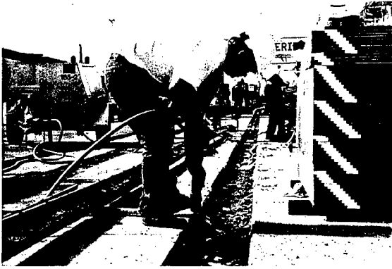
Fig. 13 – Pneumatic chipping hammer.
