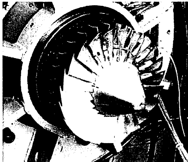
Figure 6. Rotor-Stator Assembly Prior to Casewall Installation
