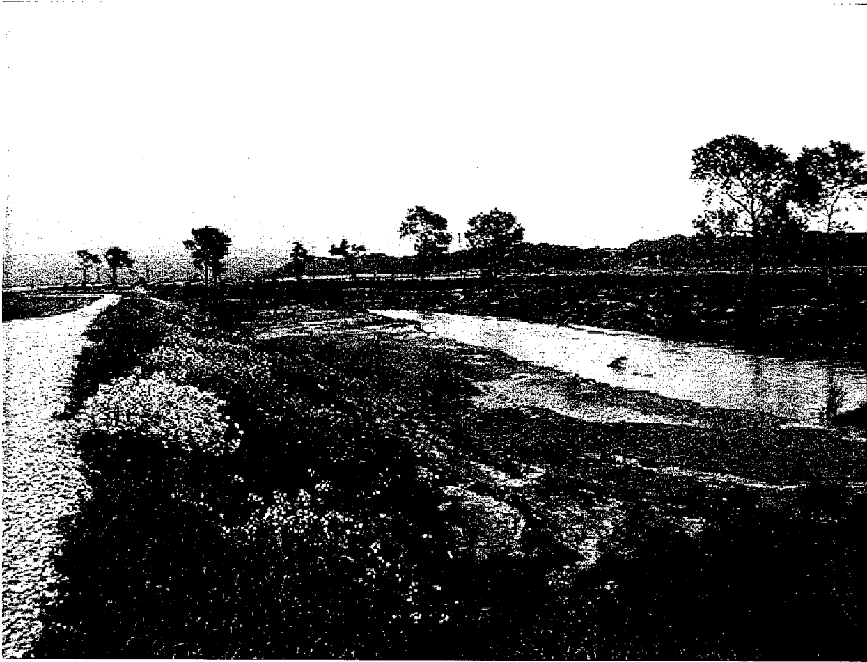
Plate 4 Upstream View of Project at Highway 1, May 1998
