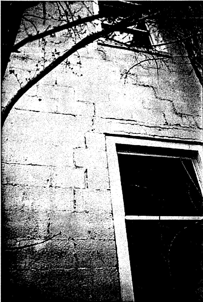
Figure 3-26. Most severe cracking at southeast window.
