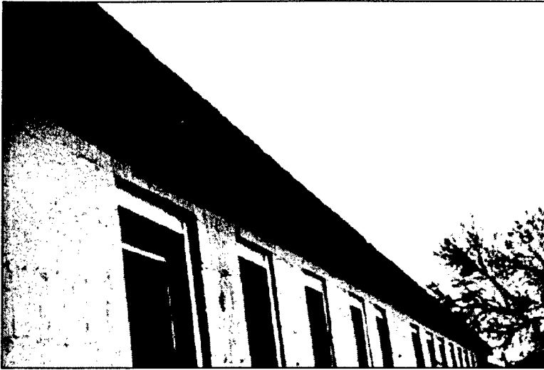
Figure 3-30. Warped fascia board.
