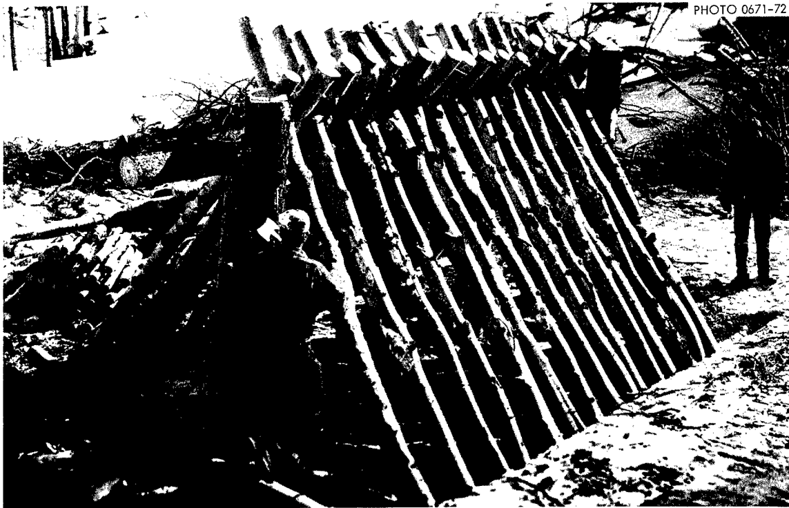
Fig. 14.4. A Russian Ridgepole Shelter, with its ridgepole resting on two logs, each wired to the tall green stumps of two fresh-cut trees 15 ft apart. All the wall poles were wired to the ridgepole and their butts were secured in two "V" trenches, each 15 ft long and about 4 in. deep. These very shallow trenches required 2½ man-hours to dig into the frozen ground with a pick. As an added strengthening, two 6½-ft-long, 8-in.-diam posts were positioned at 5-ft intervals under the ridgepole.
