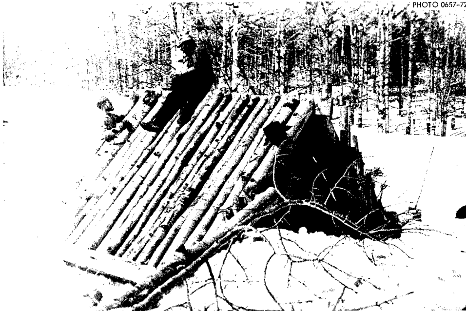
Fig. 14.7. A-Frame Log Shelter, with 45-degree sloping sides of green aspen logs, each 9 ft long, with their tops at least 4\frac{1}{2} in. in diameter and nailed to the 12-ft-long, 2 \times 8 in. ridgeboard. The butts of the 9-ft wall logs rest on the frozen ground; outward horizontal movement of the butts of the wall logs is prevented on the two sides by two 10-ft base logs. The ends of the two base logs are held in place by being fitted into deep notches cut into two 14-ft end logs. This rectangular log frame on the ground eliminates the need for time-consuming digging into frozen ground. All logs were dragged by the men through 2\frac{1}{2} -ft-deep snow an average distance of about 200 ft from where the trees were felled.
