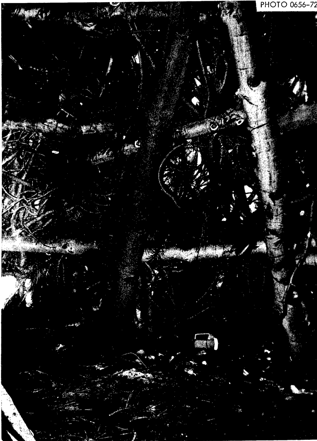
Fig. 14.3. View inside the 20-ft-diam Log-Tepee Shelter, showing three tiers of small short logs wired to the outsides of two of the twelve 17-ft main logs. The outer pine limbs were covered with 6-mil polyethylene. This shelter, large enough for at least 30 men, was built in 2.6 man-hours per occupant space. This time included the 2.7 hours it took the bulldozer to cover this 13 \frac{1}{2} -ft shelter with snow, as well as the time for its intermittent use to drag all materials to the site and to help raise the log tepee.
