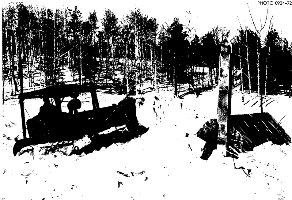
Fig. 14.8. A-Frame Log Shelter being covered with snow, after having been covered with 6-mil polyethylene. This thin plastic film kept dry free-running snow from flowing through the cracks between the logs, and prevented melted snow from dripping inside. Note the ventilation duct made of four 1 \times 8 in. boards, 8 ft long, and connected to shelter just below its top, beside its ridgeboard. The final snow covering came within 2 ft of the top of this board duct.
