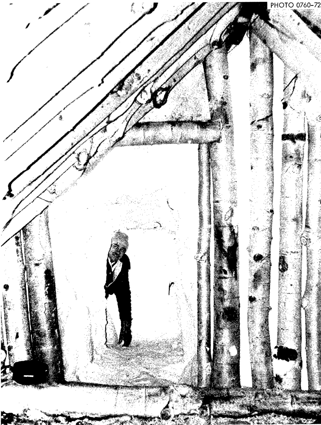
Fig. 14.9. View from inside the A-Frame Log Shelter, looking out into its entryway, a 9-ft-long snow tunnel with a 90-degree turn. This entryway has another 4 ft of snow tunnel, not shown. In the foreground is seen an end log of the rectangular log frame, with the butts of the almost vertical end-wall logs pressing against it. Outside the end-wall logs is the 6-mil polyethylene covering, which kept the bulldozer-compacted snow from entering. Snow arching, and not the strength of the polyethylene, withstood most of the pressure of the snow. To build this 10-man shelter, with all work except the snow covering done by hand, required 4.8 man-hours per space.
