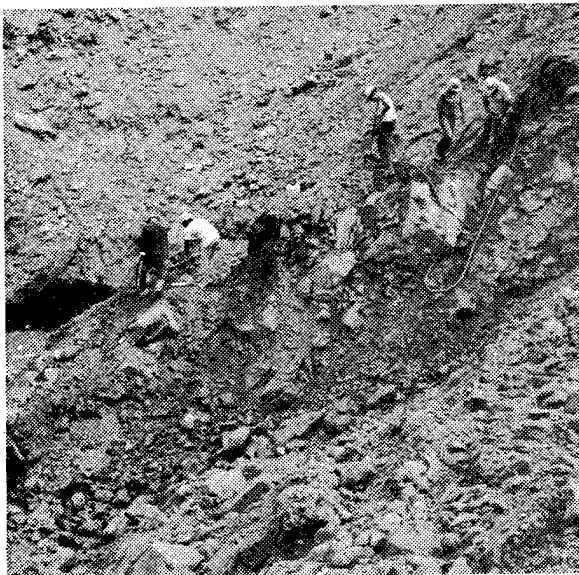
Fig. 103. Recovery of subsurface displacement pellets inside Bravo crater during postshot investigations.
