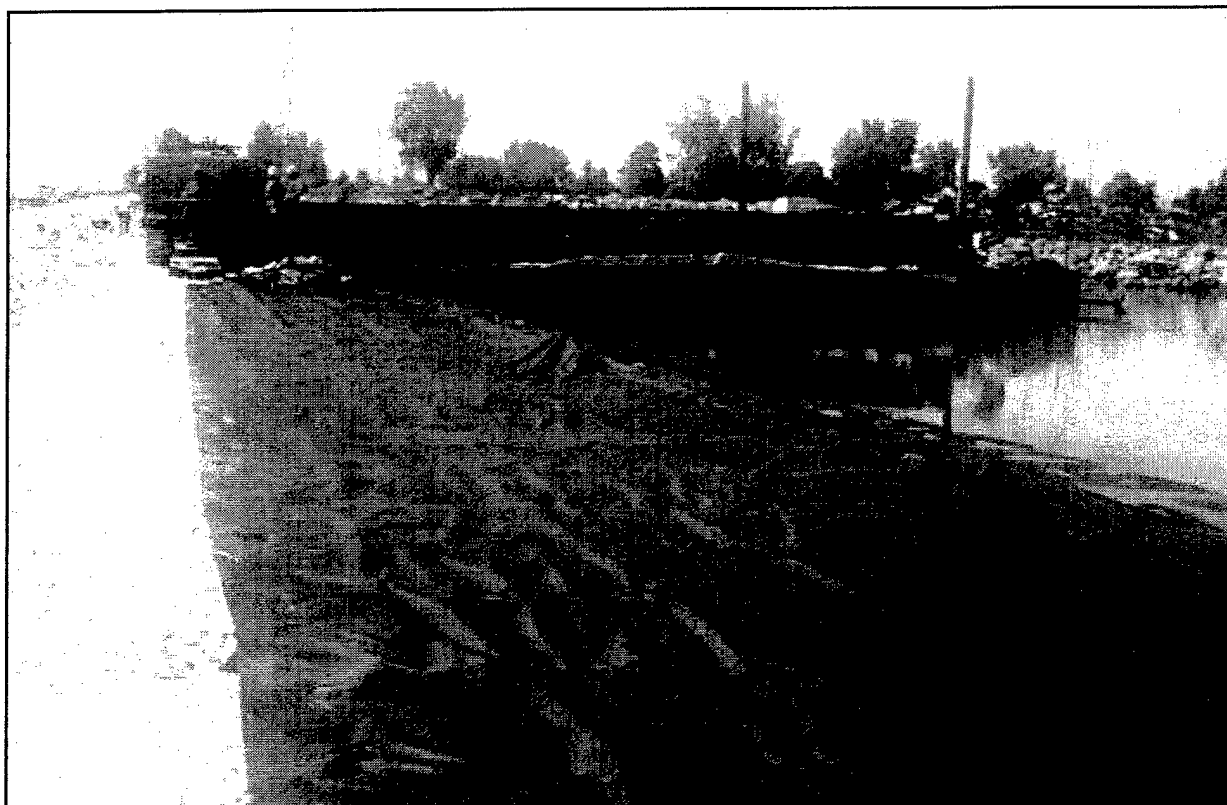
Figure 6. Chicago CDF showing placement of geomembrane on inside dike face (photo courtesy Chicago District)
