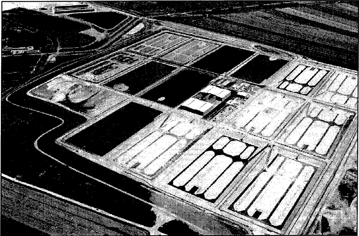
Figure 10. Aerial photo of “dewatering fields” at Bremen, Germany (PIANC)
