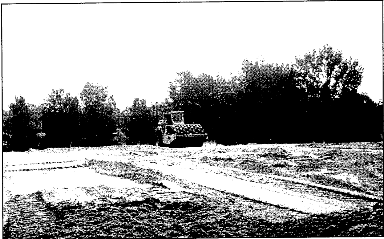
Figure 19. Michigan City CDF, showing roller compaction of cap material (photo courtesy Detroit District)
