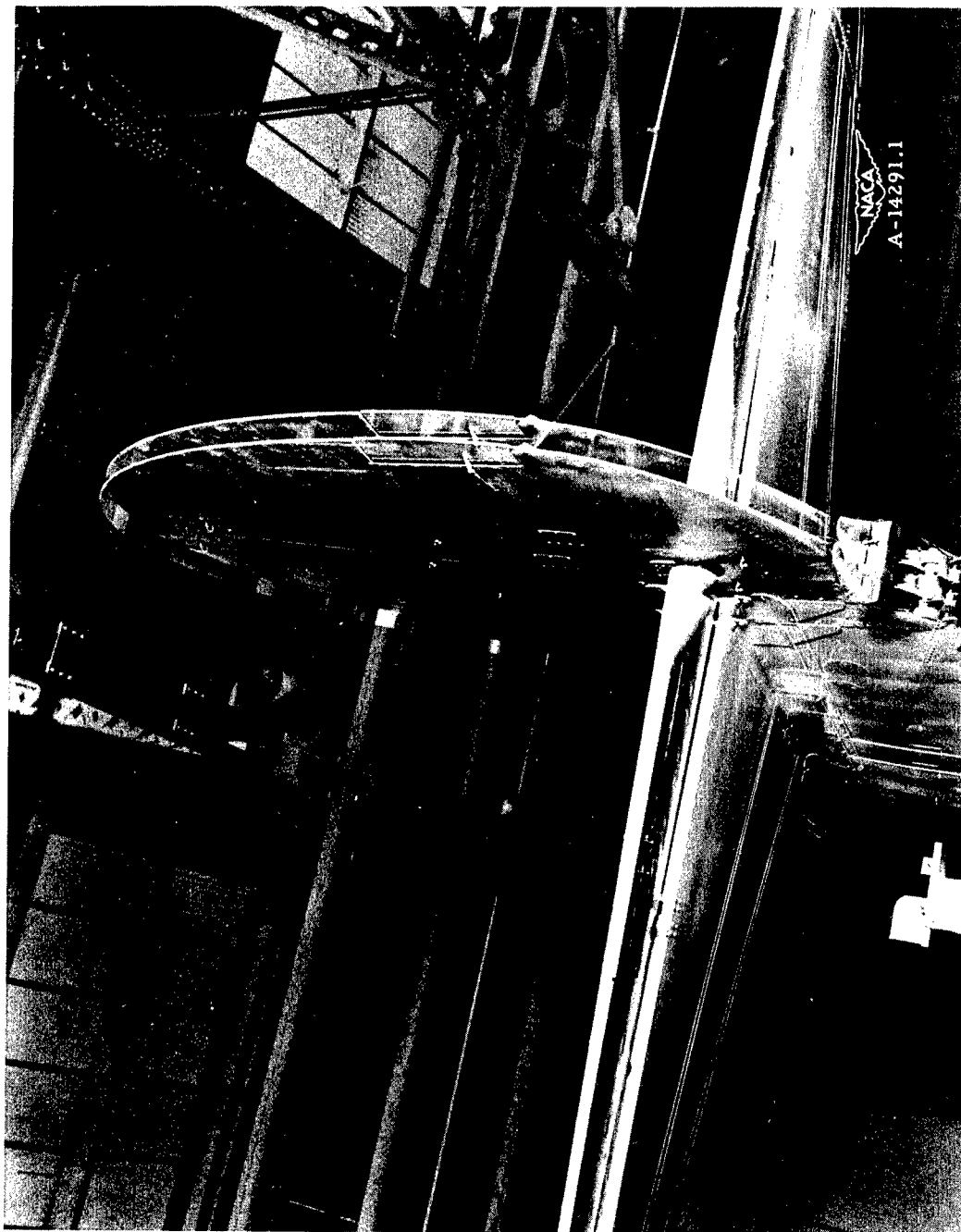
Figure 10.- Double exposure showing oscillation in yaw.
