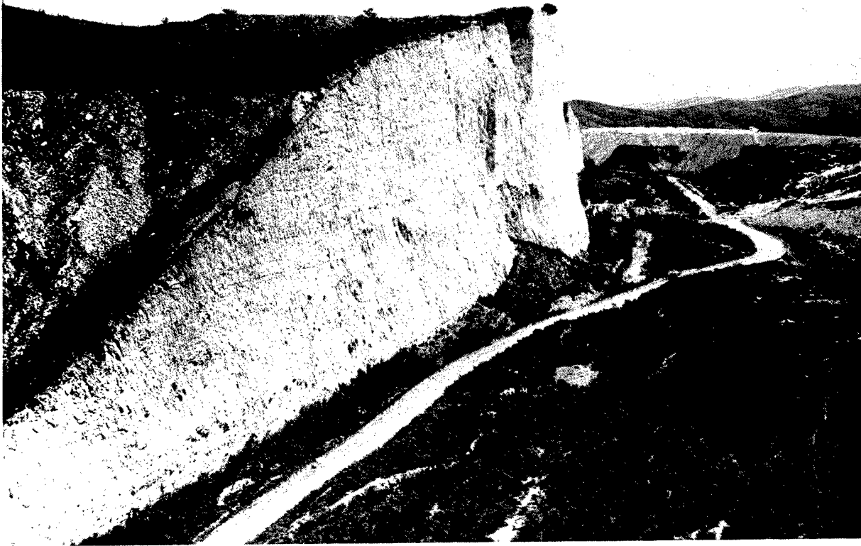
Figure 2.4 Excavated slope near Lompoc Quarry; showing near-vertical 170-foot slope in soft massive material. (Contributed by Johns-Manville Products Corporation)
