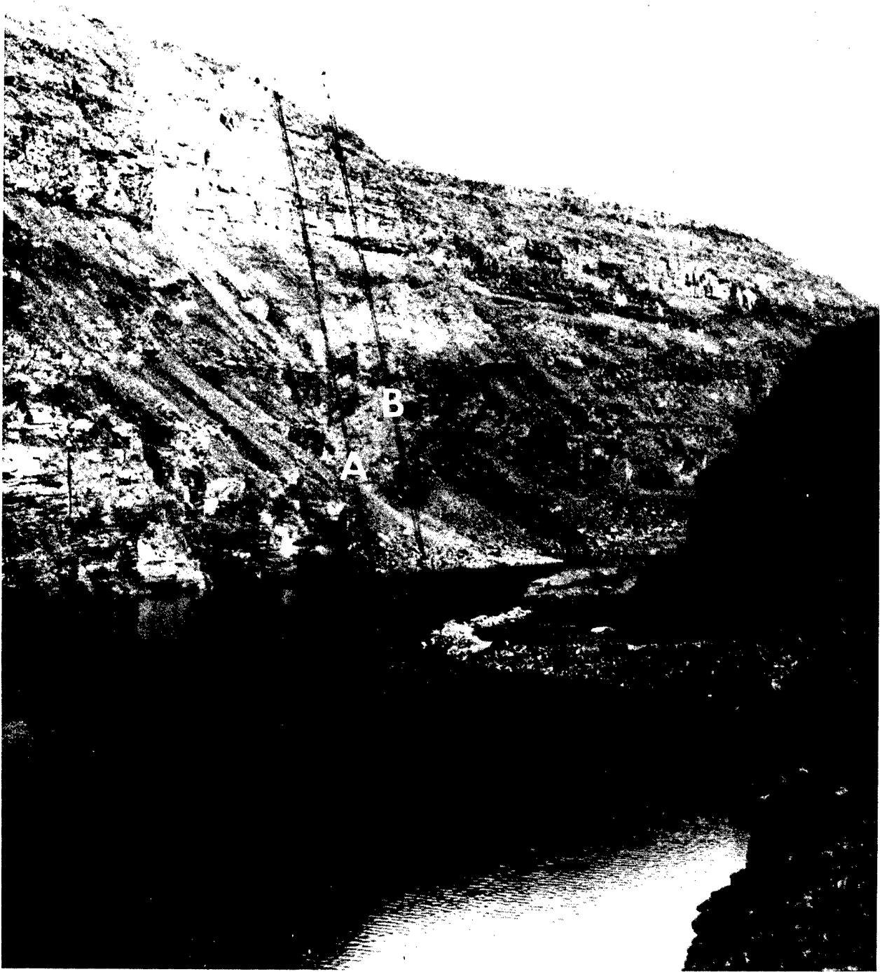
Figure A.49 Missabe Mountain Mine; view of northeastern wall, showing location of Figure A.50 sections. (Contributed by Pittsburgh Pacific Company)
