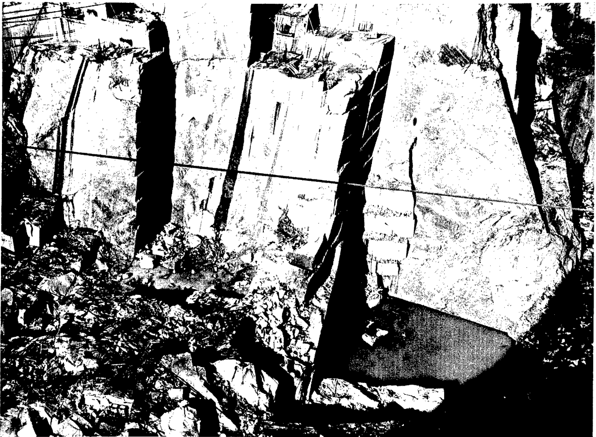
Figure 2.3 Rock of Ages Quarry; showing near-vertical slopes in hard massive rock. (Contributed by Rock of Ages Corporation)
