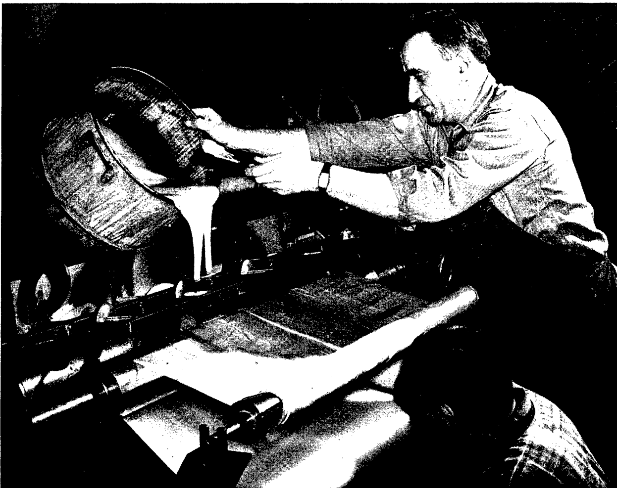
Figure 4-17. High-viscosity, laminating resin being spread on glass cloth with a machine spreader employing a resin-coated roller as an adapter to a conventional adhesive spreader.
