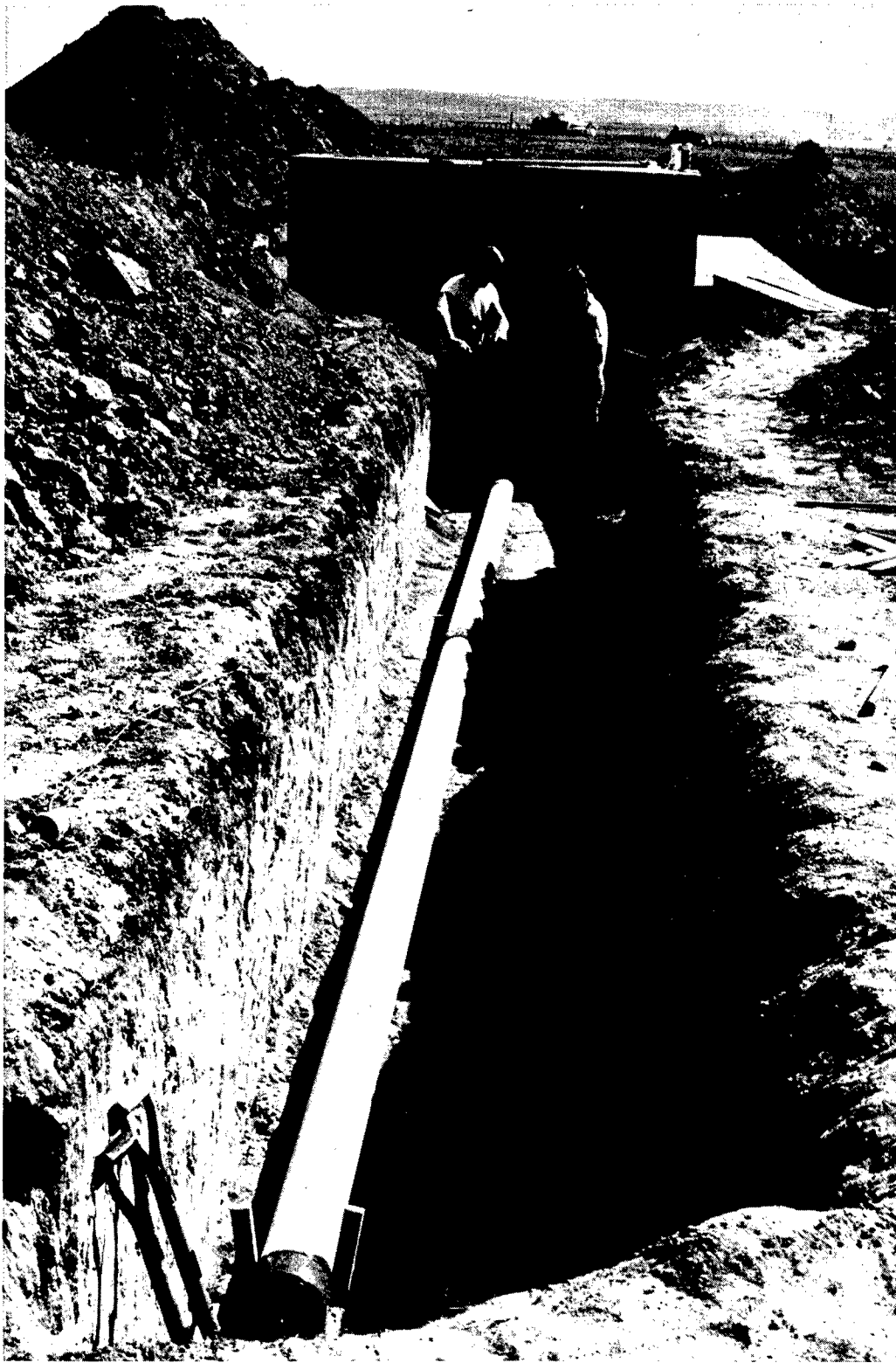
Figure 17. --Installation of the PVC conduit.
