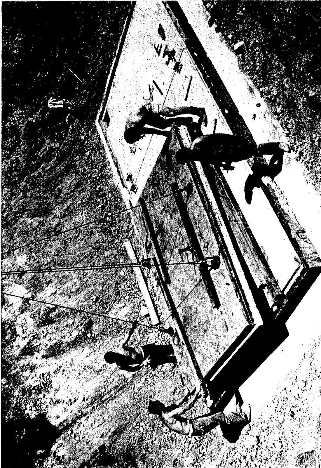
Figure 5. --Assembly of Manhole (page 2 of 10).
