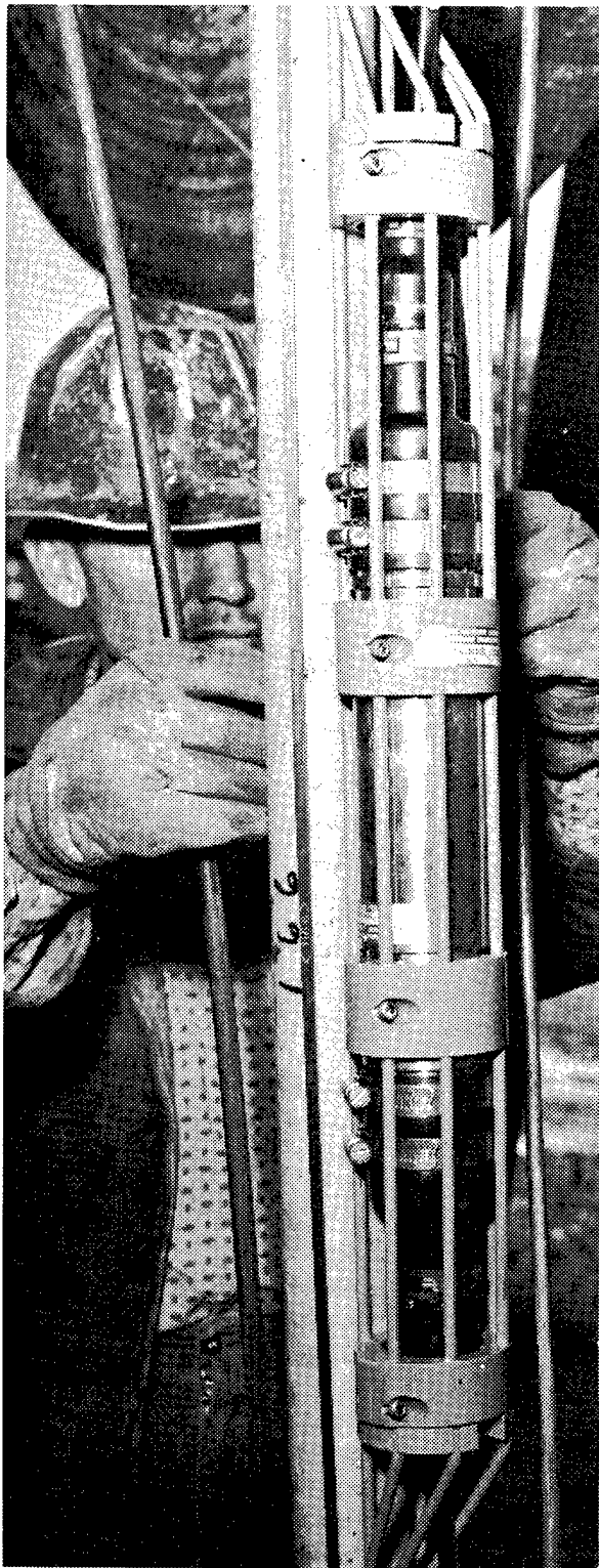
Fig. 3. Instrument being lowered in hole GB-1. Grout was pumped through the fiberglass pipe to which the instrument is attached to provide coupling with the formation.
