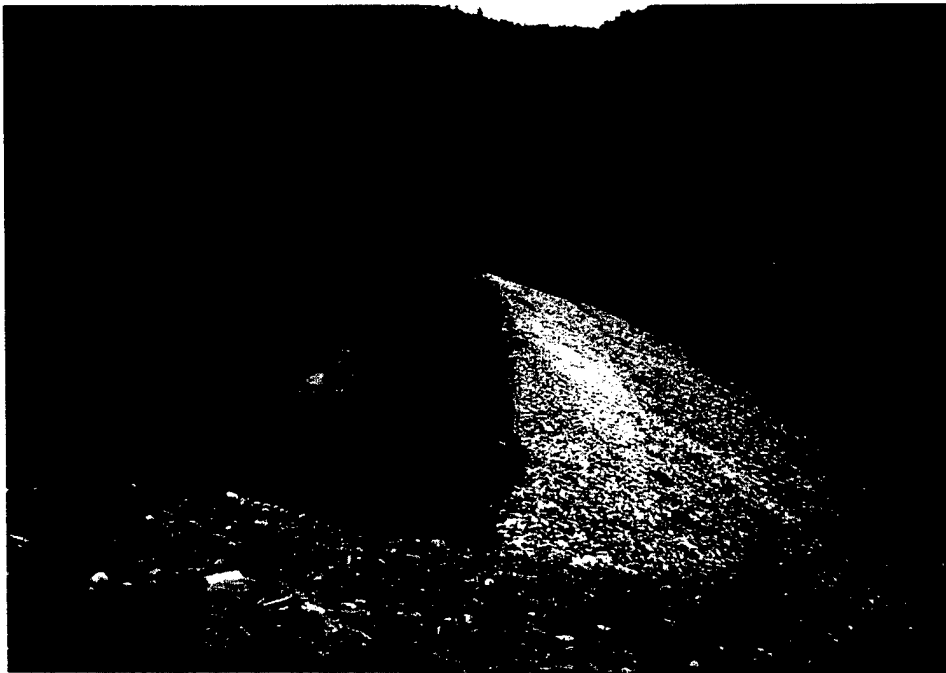
PHOTO E-6: Upper level of upstream impervious blanket. Note sapling at top of riprap slope.
