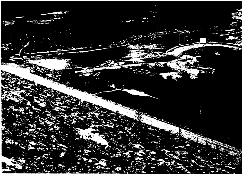
PHOTO E-10: View of seepage pool and outlet channel. Note seepage at downstream toe.
