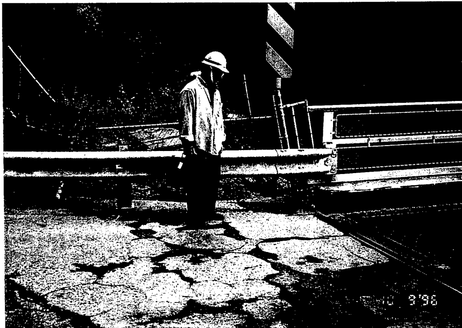
PHOTO E-16: Left side of spillway bridge. Note alligator cracking on asphalt and damaged safety fence.
