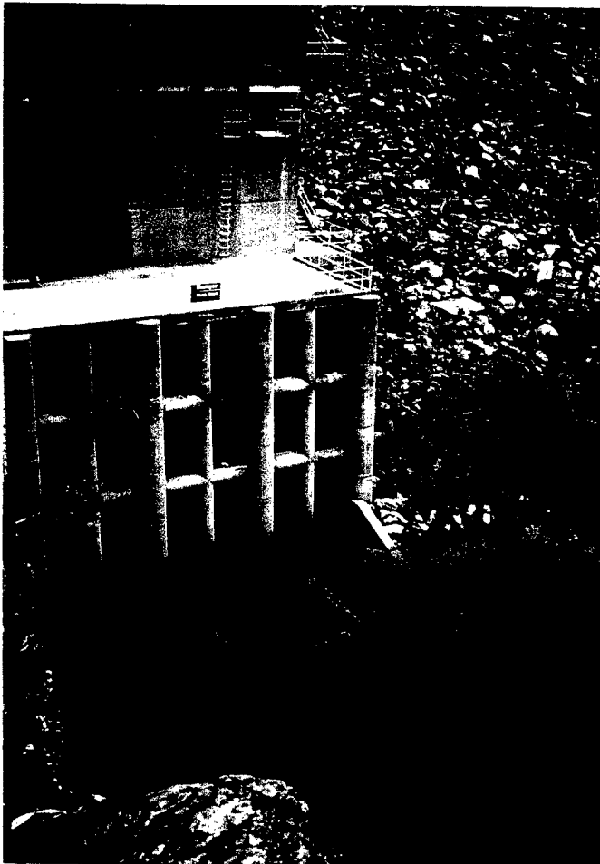
PHOTO A-14. General view of upstream control weir and trash rack.
