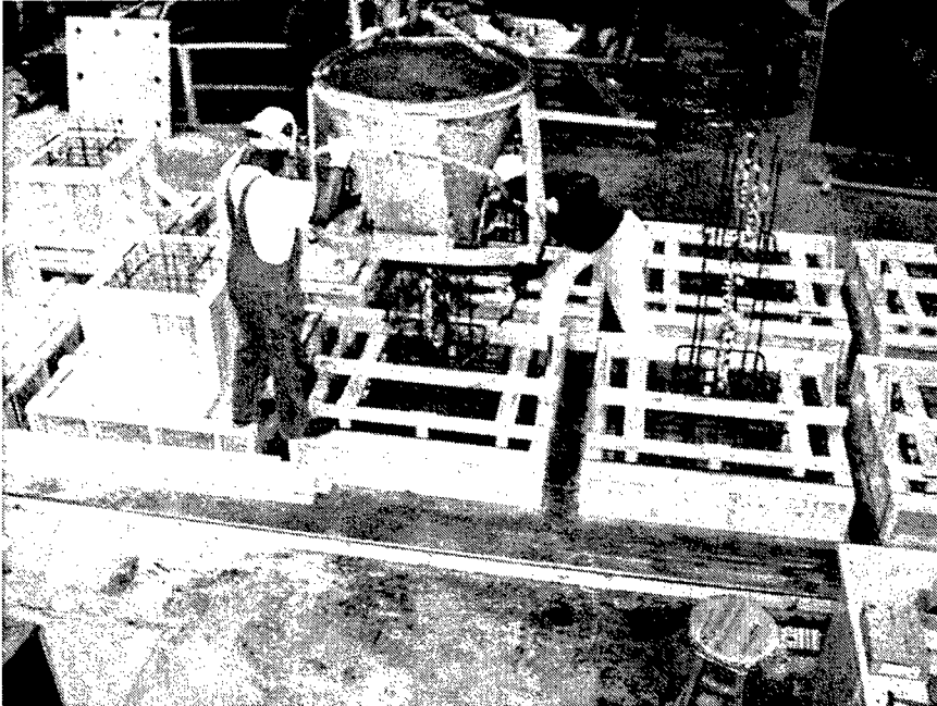
Figure 5. Base slab concrete placement
