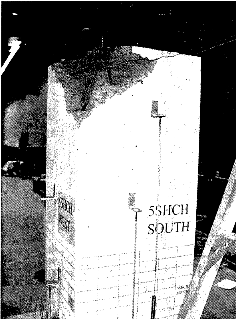
Figure 42. Damage to 5SHCH model due to accidental loading
