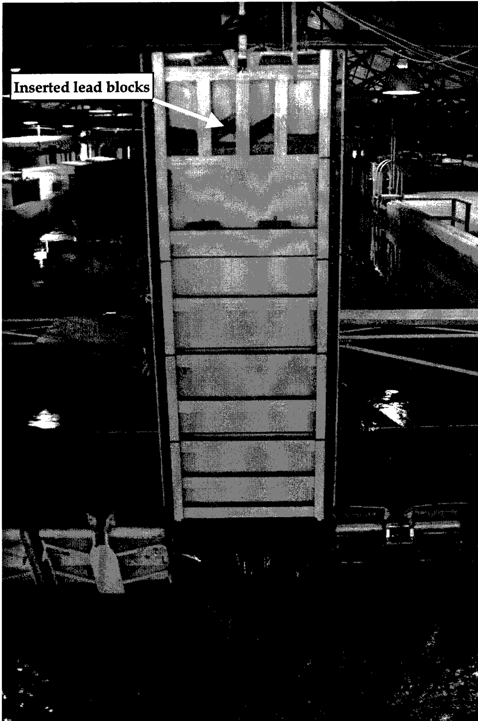
Figure 7. View from the catwalk, looking upstream at the blank in the raised position for installation. The blank has been weighted with 68.32 lb of lead positioned in the upper three channels. Headwater 301; Tailwater 294; 7-ft differential
