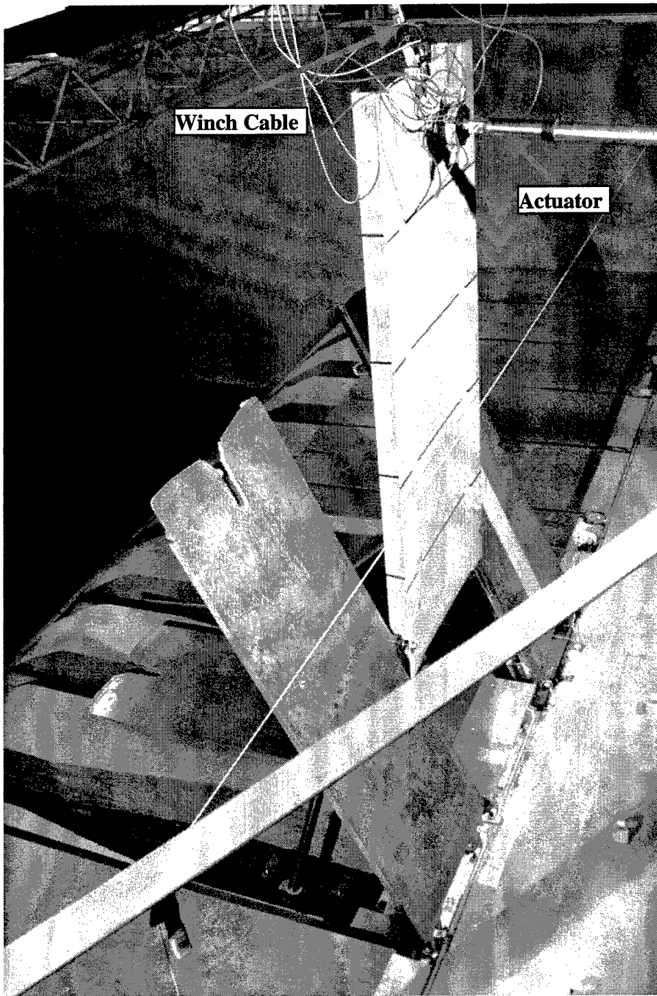
Figure 1. View from the walk, looking downstream at the wicket blank and wicket gates #4, #5, and #6. The bottom of the blank is at el 287 and at an angle of 90 deg. Dry bed photo
