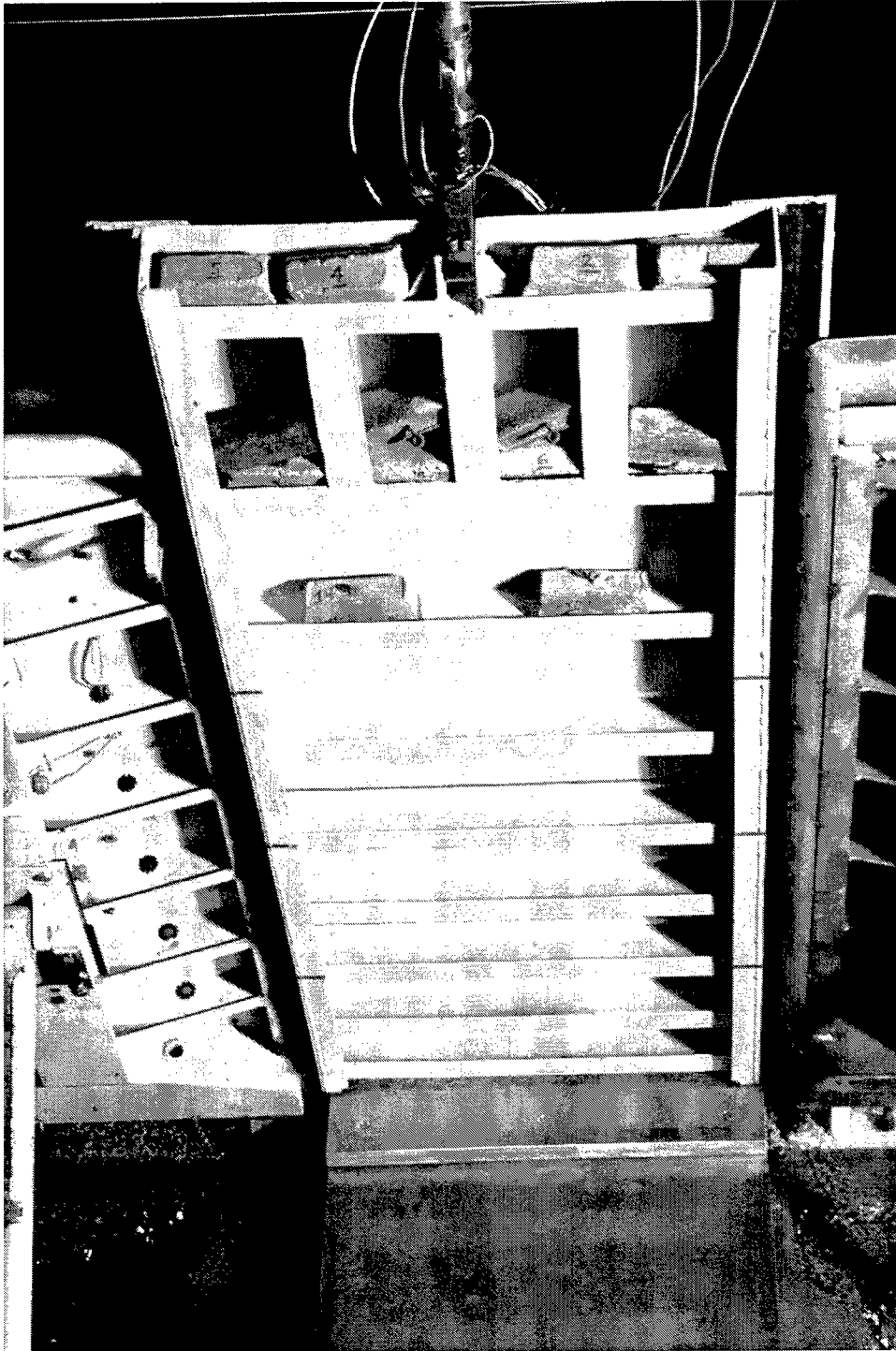
Figure 27. View from the catwalk, looking upstream at the blank seated on wicket gate #5, showing the weights located in the top three channels. Dry bed photograph
