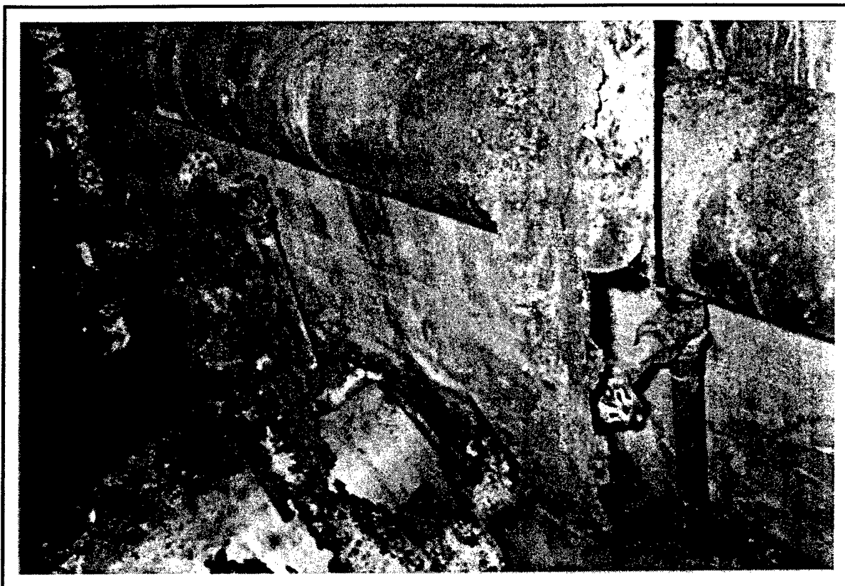
Figure 18. Corrosion scale and valved conduit in valve pit area.
