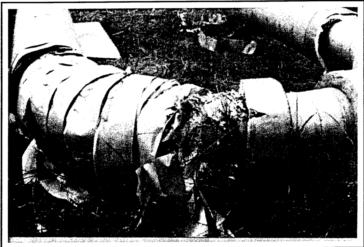
Figure 5. Steam distribution piping insulation and sheathing in poor condition.
