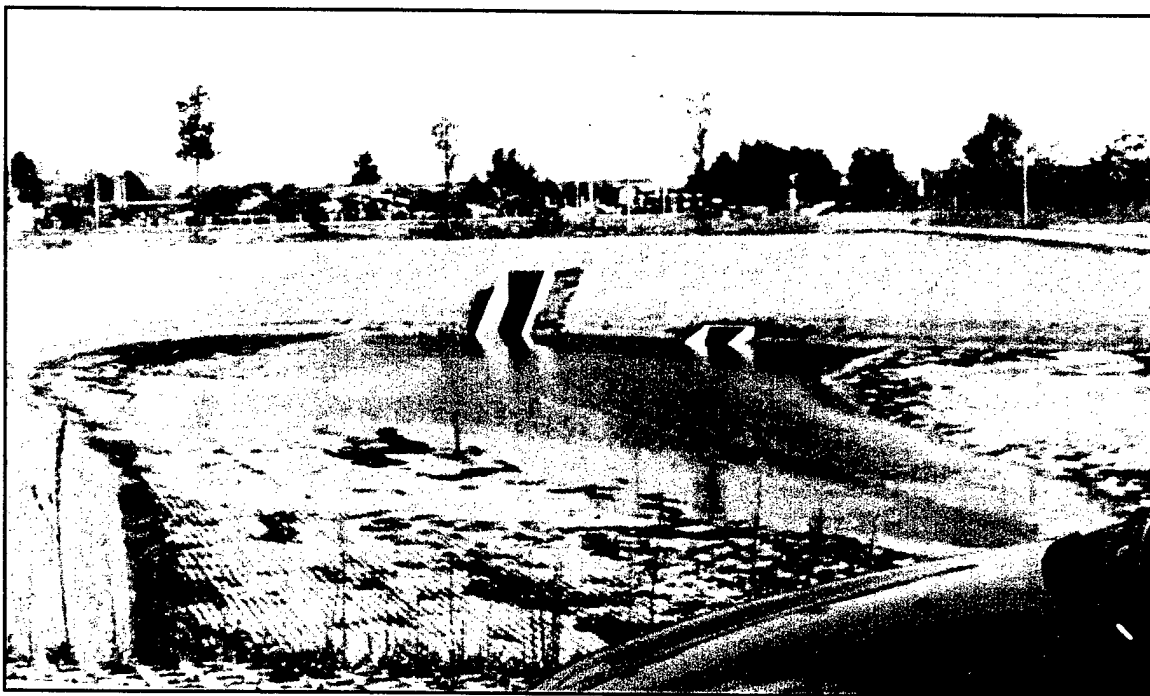
View of Newly-Completed Catchment Basin (9/98)
